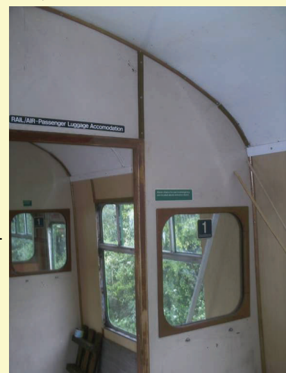
Interior restoration inside 51074 (J. Poor)
